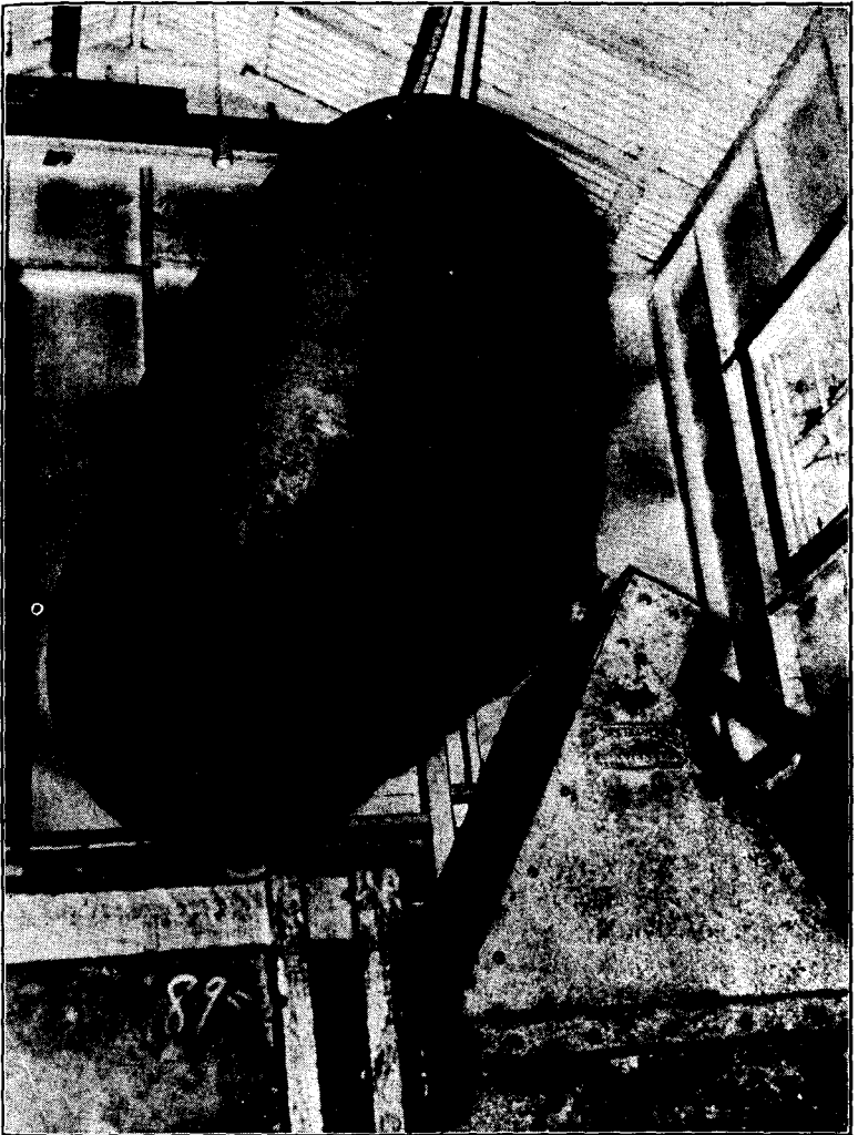
FIGURE 71. Sweetie Barrel. (Courtesy Western Cartridge Company.) The moist and mixed ingredients of bulk powder, tumbled in this apparatus, take on the form of grains. Similar equipment is used for sugar-coating pills and for applying a deterrent coating or a graphite glaze to grains of colloid smokeless powder.
